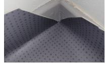
**4.** Cut section as shown, once completed open up to see perfect corner shape cut - trim edges.
